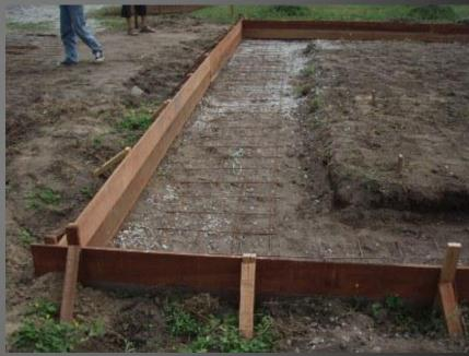
With Self Compacting High Strength Concrete we get very smooth level base that takes tile strait away, reinforcement and starter bars, we encourage the usage of bamboo to replace steel.
