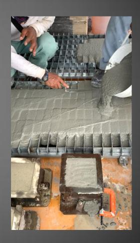
The 8 sq. ft. (0.75 m2) SIP set is made with a special RIG set which we provide and also Epoxy Solvent bonding glue with bonding agent for the cement boards
